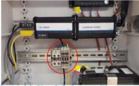
Figure 8d: Pipe & Reference IN
