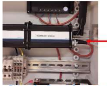
Figure 8e: Power Connected
