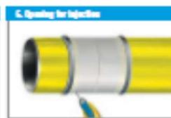
Using a carbide accessories (drill bit 5.5 mm) on the underside of the pipe near to the longitudinal point with the factory coating (approx. 2 cm), drill a hole in the coating and after the attached static mixer underneath the hole. Ensure there is enough space to manoeuvre on the ground for injection purposes.
